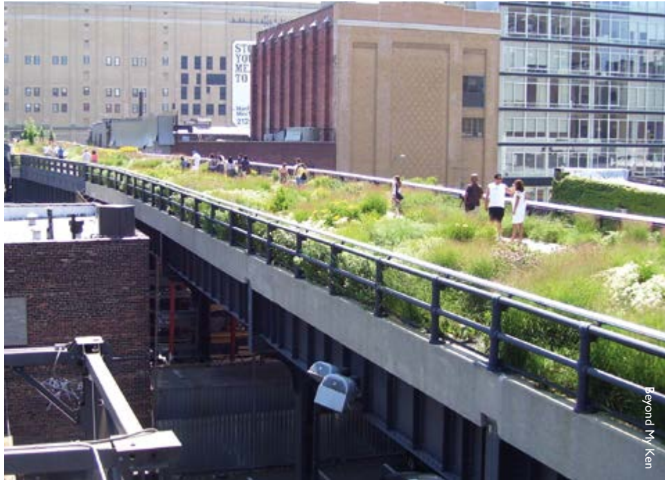
The High Line in Manhattan, New York City at West 20th Street, looking downtown (south)
